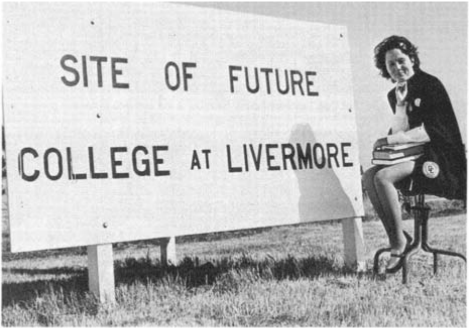
VALLEY SITE. Chabot College student Pat Alexander of Livermore perches beside a sign erected at the Livermore campus site.
