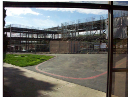
Framework of the College Center For The Arts photo taken from Building #100
